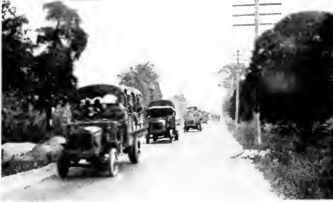
Heavy Army trucks damaged the new road surface.
